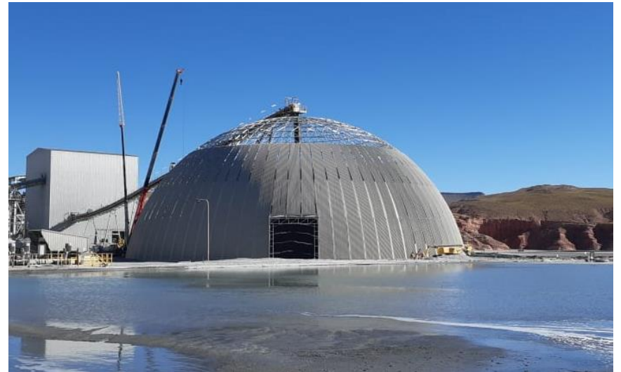
Stockpile dome construction
